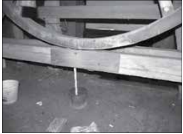
In the belfry, the rope attaches to a large wheel that provides leverage.
