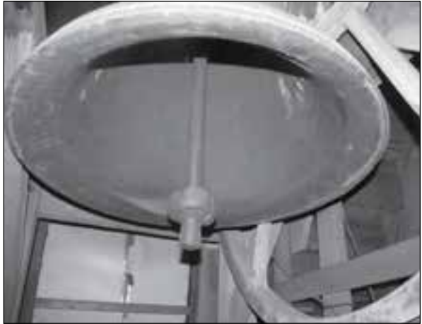
The clapper, which produces sound by striking the wall of the bell as the bell swings.
