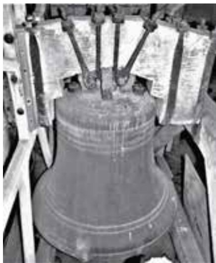
The bronze bell and its wooden headstock. Photos in this article are from the author's collection.
