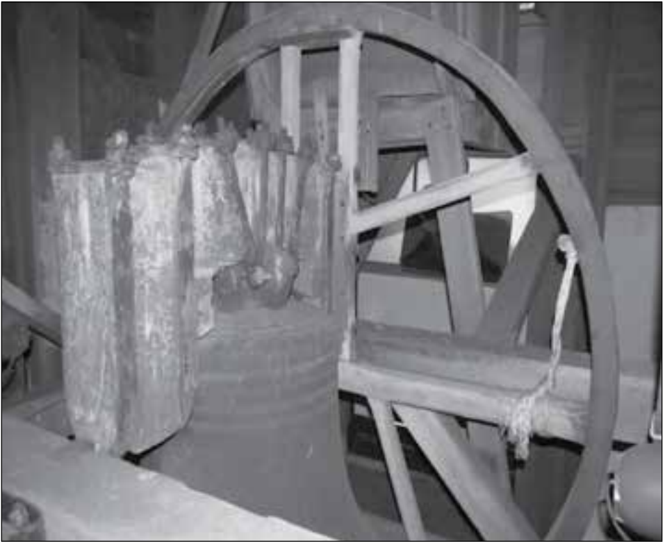
The supporting framework of the Federated Church bell, showing the large wooden wheel that provides the leverage necessary to swing the bell.
