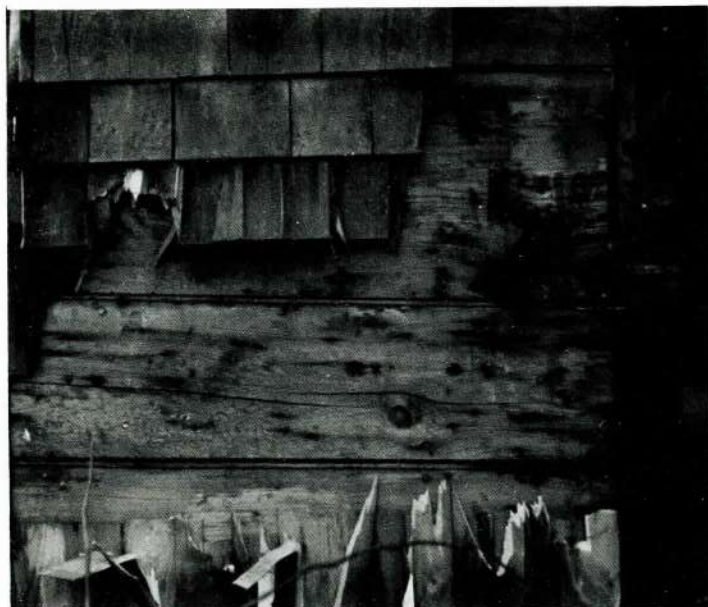
Tongue-and-groove boards cover vertical siding on Goff house.
