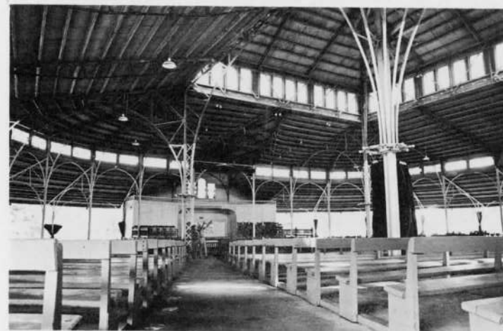
Curving gracefully, the wrought-iron frame gives a lightness to roof
