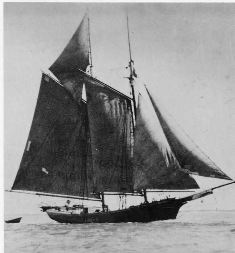
Schooner Alice S. Wentworth towing the dory and with the yawl boat on the davits. Everything set but the foretopsail and flying jib. Note the patches in the mainsail.
