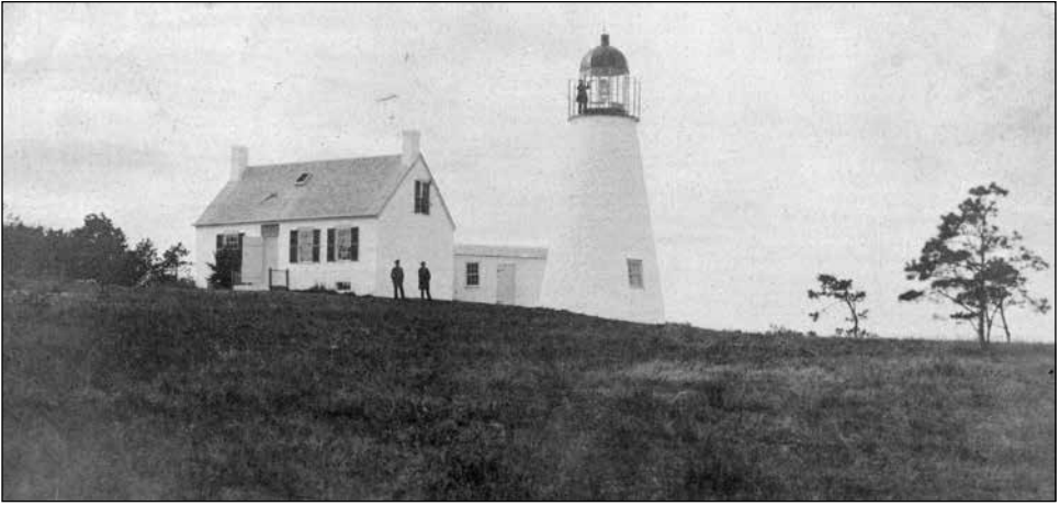
The stone tower and keeper's house at West Chop sometime between 1857 and 1863. The tall lantern with its domed roof, probably installed when the tower was moved and reassembled in 1846, was similar to those installed at Gay Head in 1854 and Cape Poge in 1857. The barrel-shaped fourth-order Fresnel lens is clearly visible inside.
