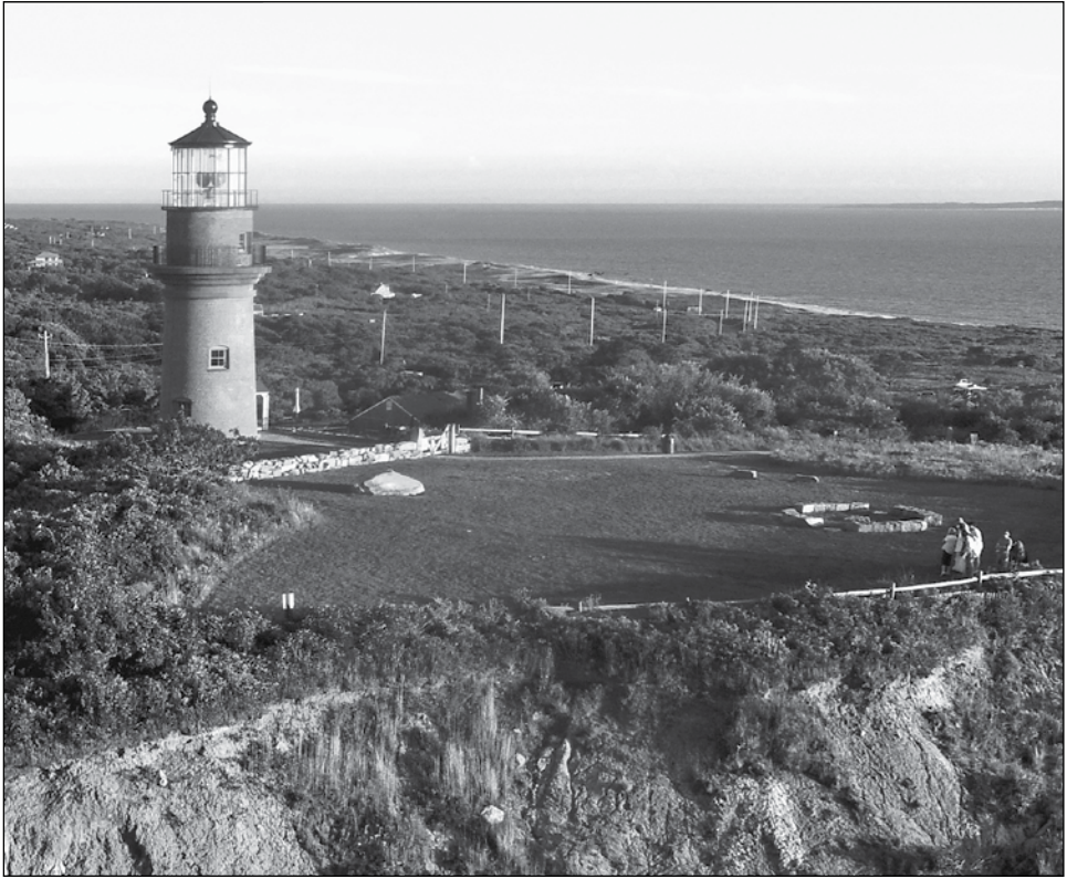
Its stone foundation settled on a new concrete base after its 2015 move inland, the Gay Head Light is expected to be safe from erosion for 150 years. The circle of stones at right marks its pre-move position at the edge of the cliff. —Photograph by, and courtesy of, Denys Wortman.
