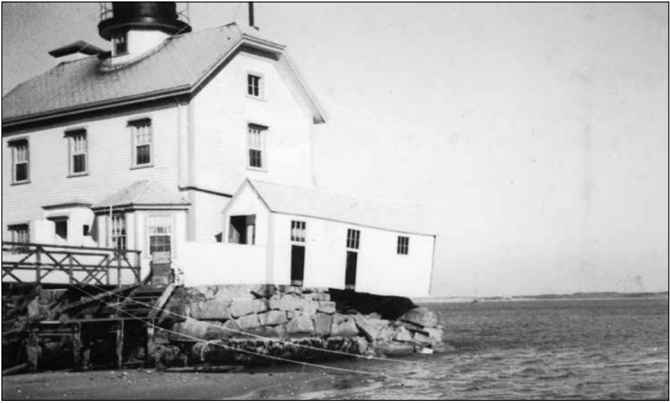
Damage done to the lighthouse's foundation by the 1938 Hurricane was relatively minor, but the repairs it required delayed replacement of the lighthouse by several months.
