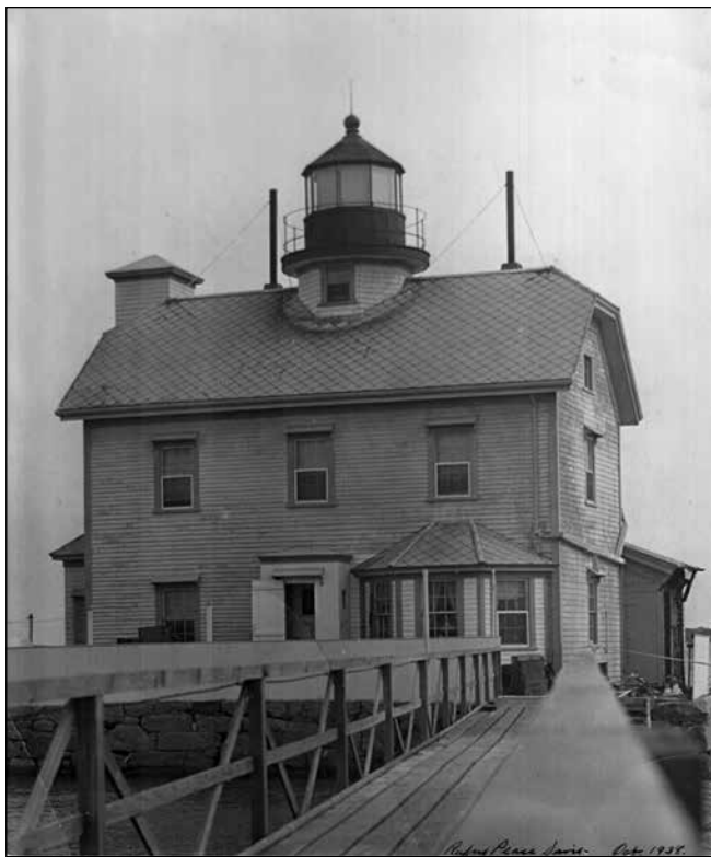
The Edgartown Harbor Light, more than a century old when this photo was taken in early September 1938, looks solid and well-kept, but it suffered from leaks, rot, and vermin. The decision to demolish and replace it had already been made.
