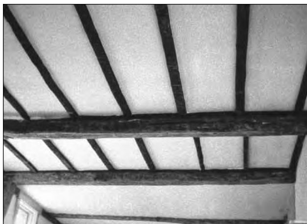
Figure 6. The ceiling of John and Elizabeth Mayhew’s half-house kitchen showing saw marks and uneven cutting of the early pit-sawn joist (This area restored by Jonathan Scott and crew, 1986).
