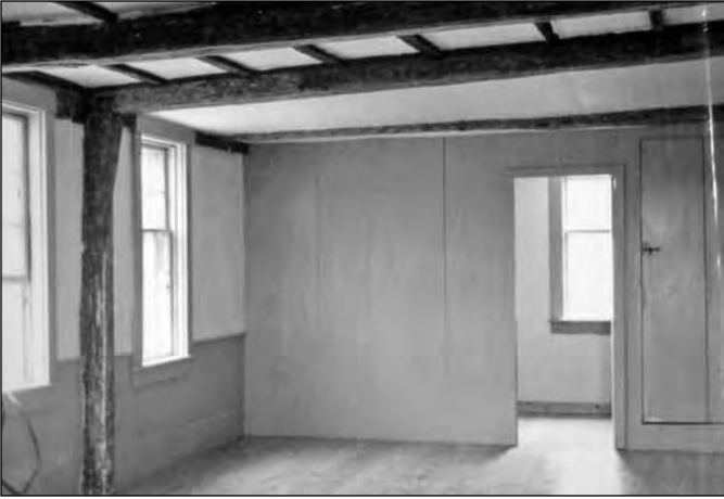
Figure 9. Looking from the pit-sawn joist and flared post of John Mayhew's half-house kitchen toward the new eastern part added by Russell Hancock. Through the open door is the borning room where Deborah may have given birth to her seven children (Restoration by Jonathan Scott and crew, 1986).
