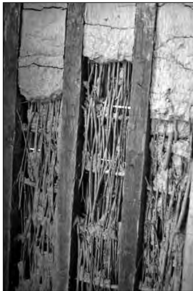
Figure 3. Wall with wattle and daub from Plimoth Plantation.
