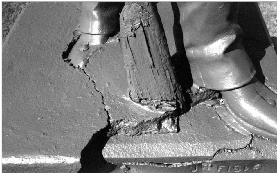
Before restoration, the statue's entire cast-iron base was failing.
