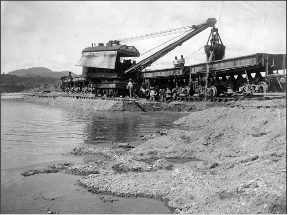
Gathering gravel with orange peel crane from Changres River, January 1912. — MVM collections
