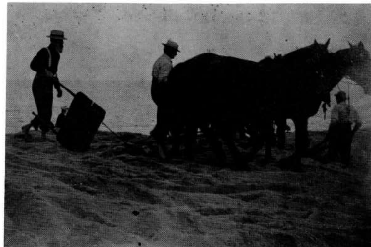
The latest word in earth-moving equipment in the 1890s was a simple homemade wooden drag, being held upright here by West Tisbury's Torrey Hancock.
