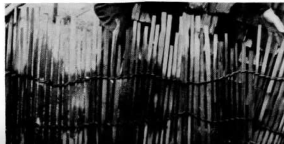
Pine-root lacing holds the slats together. Below, the leader that runs from the heart up onto the beach.
