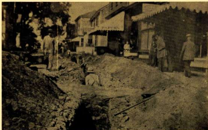
The Edgartown Engine Company was renamed the Edgartown Fire Department in 1906 when the Water Company installed hydrants, making pumpers, or "engines" as they were called, less important. Here, Main Street is being dug up for the new water mains in 1906.
