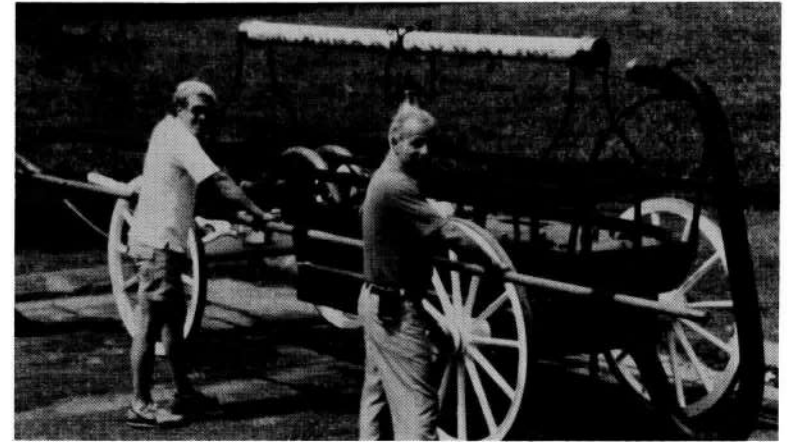
In 1984, the old Button hand pumper, shown here with firemen manning one of the brakes, was rebuilt by the Edgartown Fire Department.
