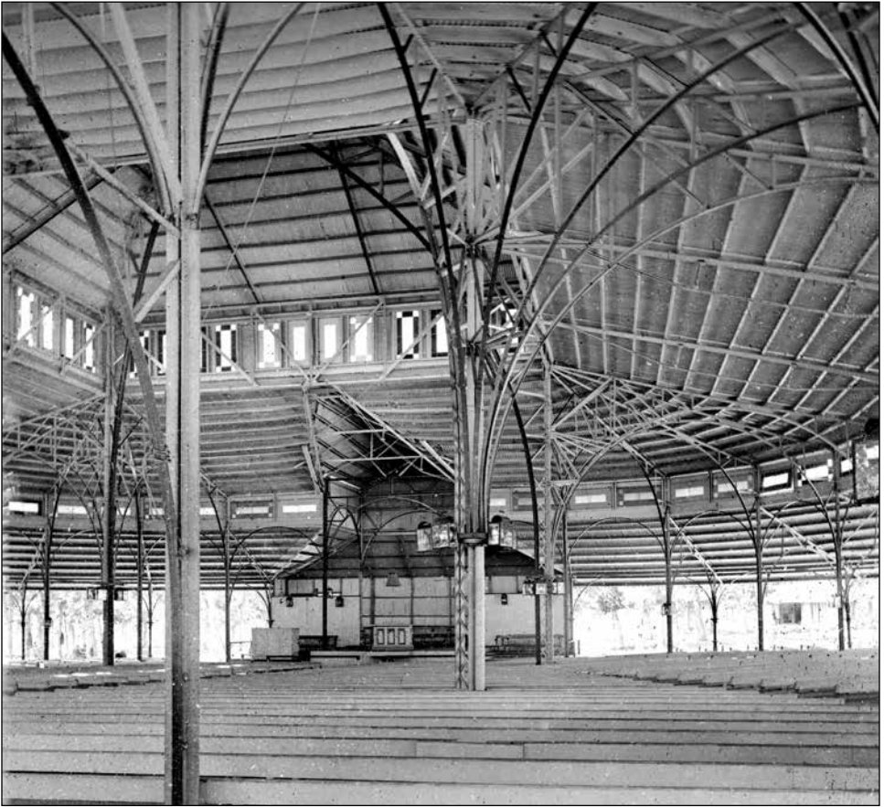
Fig. 3—The interior of the Tabernacle taken shortly after it was constructed. Note the wooden purlins in place between the iron trusses to support the corrugated roofs. MVM Photo Collection.
