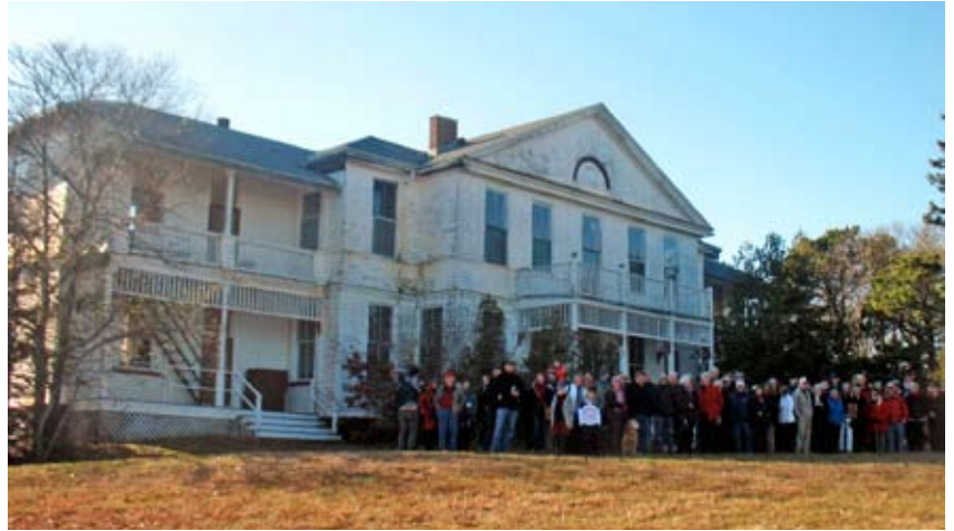
New Museum Property in Vineyard Haven on the day of the first Community Open House in December 2011.
